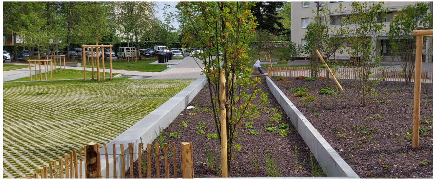
Surface rainwater management.
