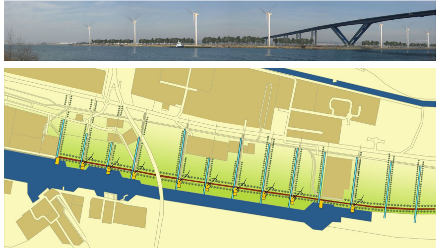
The setting-up of wind turbines is the tool to create the infrastructure of a development
