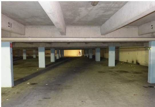
Inside of the underground parking
